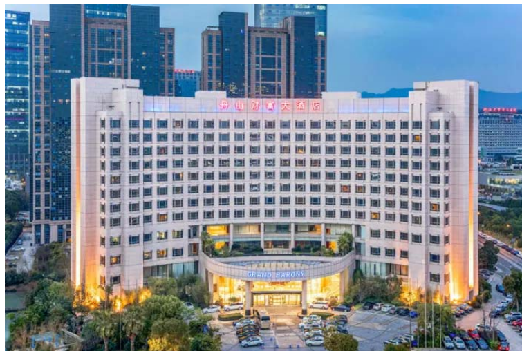
Figure 1 Zhoushan Caifu Hotel
